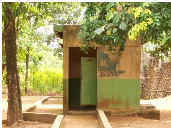
Photograph 7 Adequately Lit and Ventilated Latrines Used by Students
